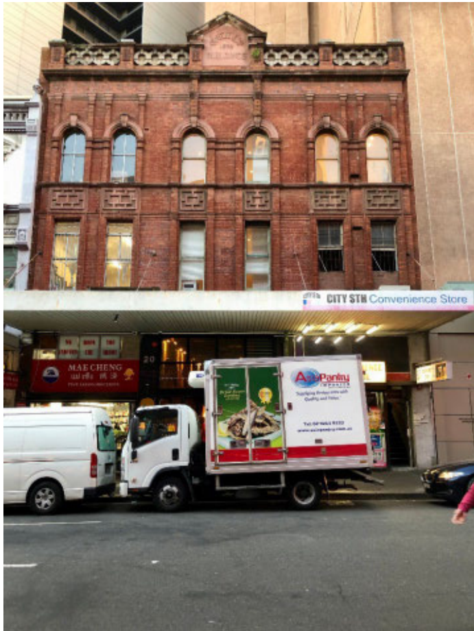
Figure 4.21 The 1890s building at 18–22 Campbell Street, Haymarket. Wing Sang occupied this building from 1895. (Source: The China–Australia Heritage Corridor)
